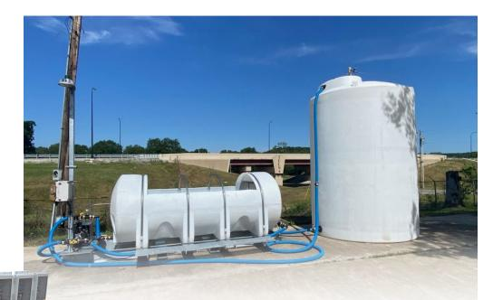
**Brine Production System** (BPS) lowers operation costs by using readily available materials; granular salt and tap water. They are capable of producing up to 5,000 gallons of brine per hour, depending on the water source.
